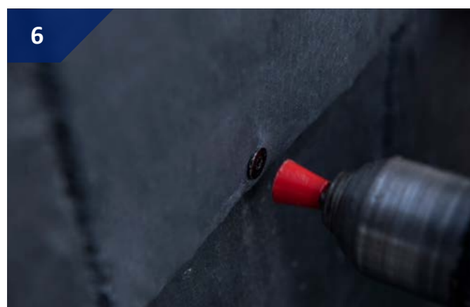
Fix the slate with 2 new screws lacquered in black
