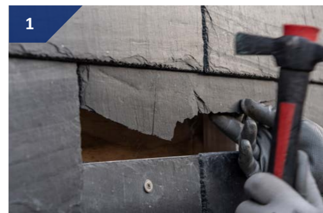
1 Break the damaged slate
