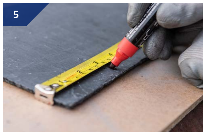
Drill a hole in each corner of the slate with a \varnothing 3/16" drill • 3/4" from the bottom • 3" from the lateral (right and left)
