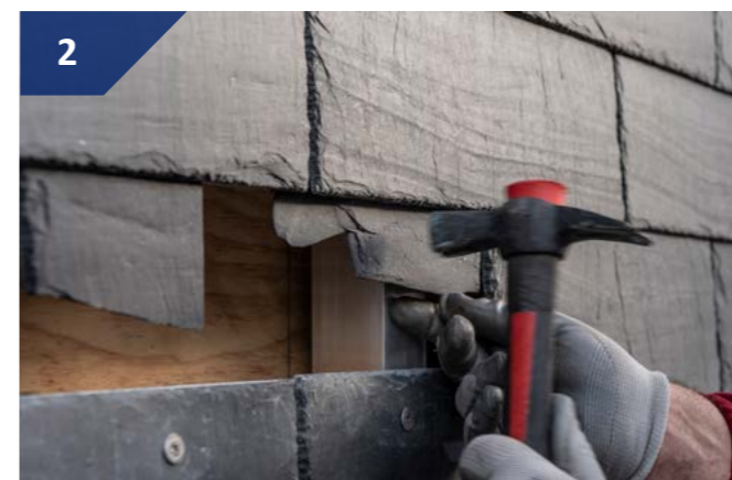
2 With a hammer, remove the broken pieces of the slate
