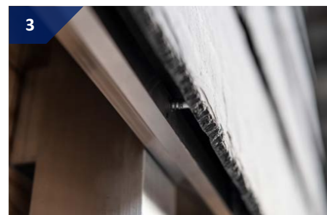
3 Cut the screws holding the broken slate with the saw
