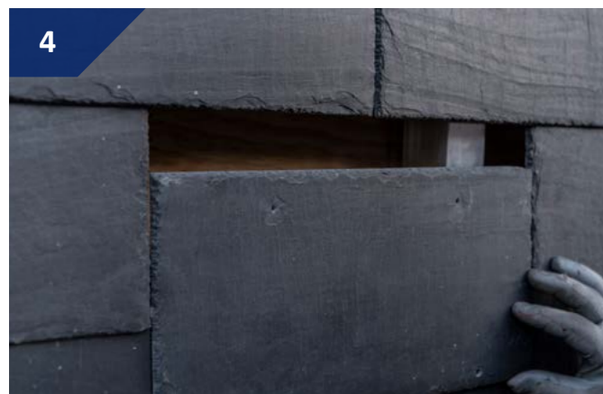
Place the new slate with the help of a hammer
